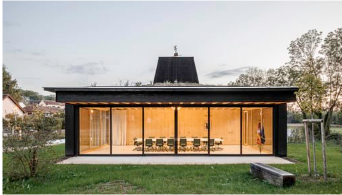
New Town Hall of Scharrachbergheim. Young architect/designer contributor: Pascal Philbert, AI Pepe Architects, France. Image credit: 11h45 – Florent Michel
